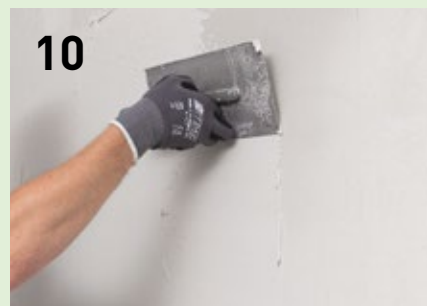
10 Mix iQ Fill fine plaster and fill. When hardened, the plaster is permeable and water-resistant.
