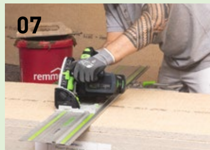
07 Cut the wall connection panels to size using the Festool TSC 55 and guide rails. Where necessary, sand down any protruding joints with the ETS EC 150/5.
