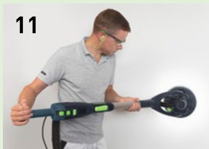
11 Sand down the filled wall using the Festool PLANEX LHS 2 225 long-reach sander and the Granat Net P120-P180 abrasive.
