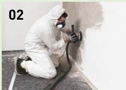
02 Remove defective areas of plaster and old coatings using the renovation miller or the surface-restoration grinder.
