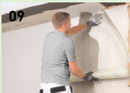
09 Using the smoother, integrate reinforcement fabric in the reinforcing mortar using overlapping, crease-free vertical strokes.
