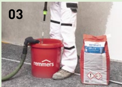
03 Mix PP Fix, an adhesive mortar for mould remediation, using the Festool MX 1200 stirrer and the HS3L mixing container.
