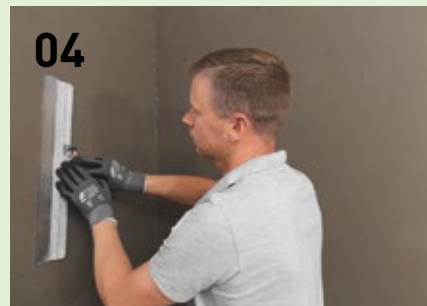
04 Level off (up to 8 mm) the substructure using adhesive mortar PP Fix and a wide filling trowel.
