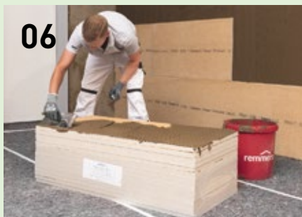
06 For full-surface adhesion of insulation panels, PP Fix is applied to the wall and panel using a toothed trowel.
