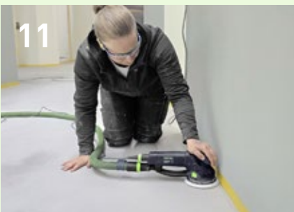
Sand the entire floor surface: cover wide areas using a Trio disc sander and work in the edges and hard-to-reach places with the ROTEX RO 150 or RO 90.
