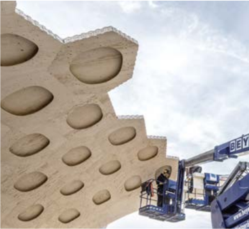
→ The hollow tile segments were partially pre-assembled and put together on site without substructures or a support frame.
