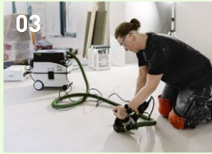
Cut cracks in the screed or clogged expansion joints using the DSC AG 125 FH freehand cutting system.
