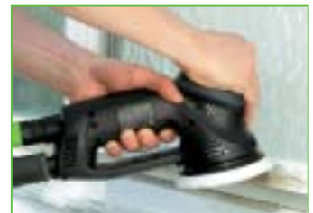
Coarse sanding of weatherboards.
